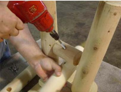
9. Use 3 3/8” lag bolt to secure the seat brace to the leg brace, as shown in this photo series.
