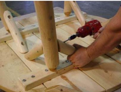
3. Use 2 ½” lag bolts to secure the 9” leg braces to the table legs and to the table underlay (as shown in these two photos).
