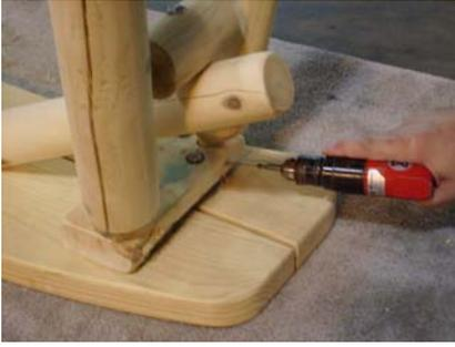
10. Use 2 ½” screws to secure the doweled end of each bench leg to the seat underlay.
