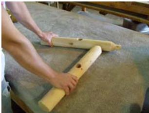
1. Insert doweled end of single-hole leg piece into double-hole leg piece. Be sure that both remaining holes are facing the same direction (as shown). Repeat process with remaining two leg pieces.
